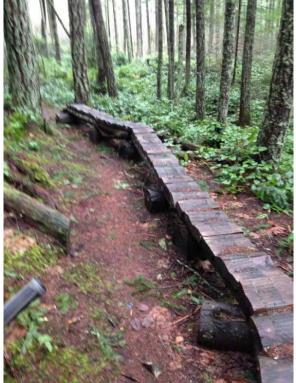
This technical trail feature is located on the "Chicken Run" trail. This structure has been considered "Ride-able but unsafe" due to the exposed rotting wood, combined with an off camber surface.
