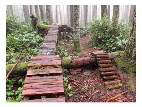
These wood structures are located on the trail "Chicken Run 1". These structures are marked as "Ride-able but unsafe due to protruding nails, and old slippery woodwork.
