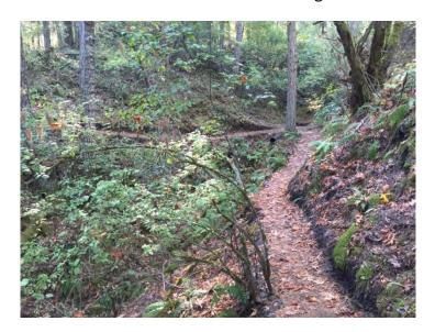
The photo at left was taken on the trail "A Grand Traverse." This recently built climbing trail was rated as being in excellent condition. This bench cut trail was built to shed water naturally by following the up and down contour of the land. At major stream crossings large culverts with sinks have been installed to capture and drain the water.
