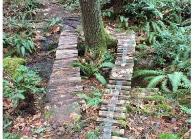
This dual bridge feature is located on a popular trail called "Danalyzer". It is considered "ride-able but unsafe" due to aging wet wood and on the left, a lack of mesh for grip.
